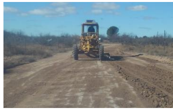
Grading East Hunt Road & Santa Cruz Road
