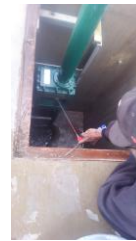
Preventive maintenance on our Muffin Monster to keep our sewers in good working order!
