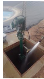
Preventive maintenance on our Muffin Monster to keep our sewers in good working order!
